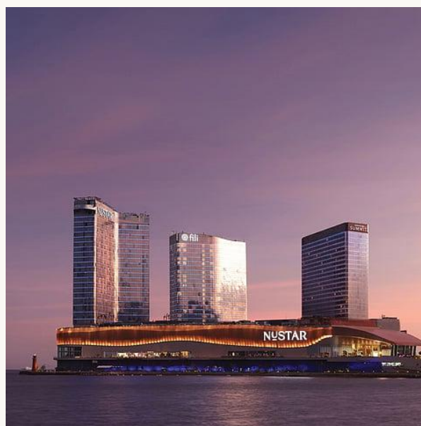
FIG. 01 • A COASTAL CEBU HIGH-RISE — NUSTAR RESORT & CASINO AT SOUTH ROAD PROPERTIES, CEBU CITY. THE ENVELOPE CARRIES THE FULL TYPHOON-SEASON LOADING OF THE VISAYAS STRAITS.
