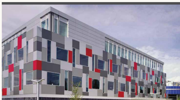
FIG. 01 • A MINERAL-CORE ALUMINIUM COMPOSITE PANEL INSTALLED AS TOWER CLADDING. THE PANEL THAT BEHAVES AS FIRE-RETARDANT IN REAL CONDITIONS IS THE PANEL THAT WAS SPECIFIED TO.
