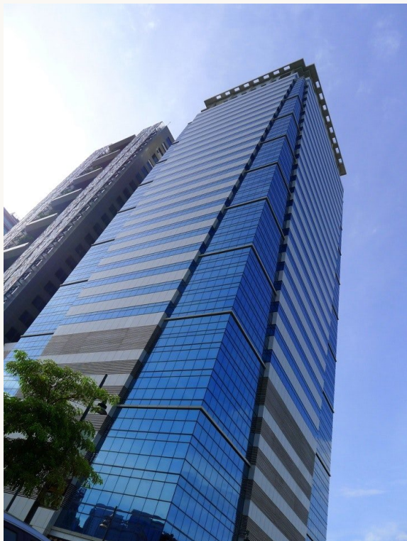
FIG. 02 • ECO TOWER, BONIFACIO GLOBAL CITY — A UNITIZED CURTAIN WALL OFFICE ENVELOPE, PHOTOGRAPHED FROM THE STREET AS THE SYSTEM READS AGAINST THE SKY.
